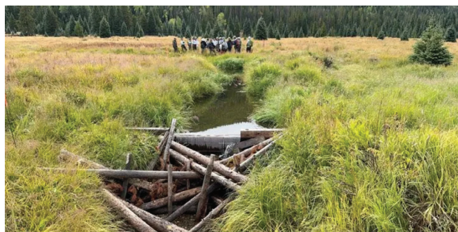
One of the artificial dam structures built along Beaver Creek to begin restoring wetlands and attracting beavers and willow growth back to Kawuneeche Valley. (Kawuneeche Valley Restoration Collaborative)
