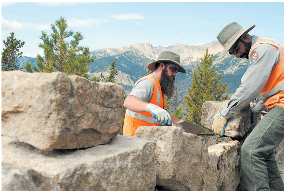
In this Tuesday, Aug. 23, 2016 photo, Kaeli Roman, right, and Louis Browning, skilled masons who work for Rocky Mountain National Park, Colo., replace one rock at a time on a historic wall the Civilian Conservation Corps built by hand about 70 years ago. This summer, he and Browning have teamed up on a 150-foot stretch of wall along Trail Ridge Road, an area that overlooks the Never Summer Range, the Kawuneeche Valley and the headwaters of the Colorado River. (Pamela Johnson/Loveland Daily Reporter-Herald via AP)
